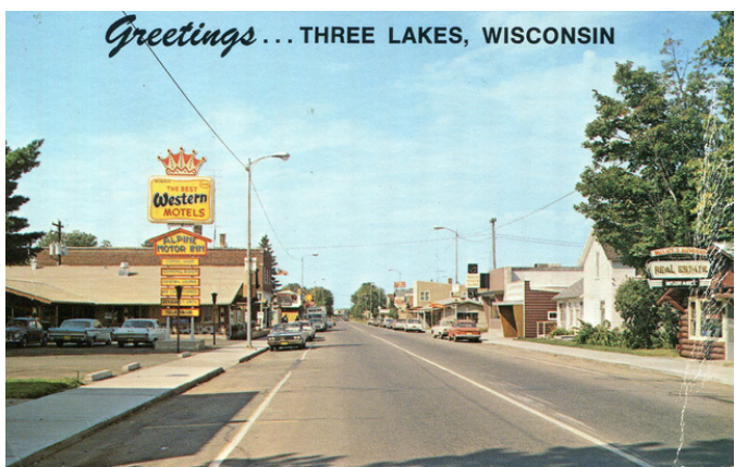
In the late 1960's, the looks of the iconic corner changed as the original building was torn down and replaced by the Best Western Alpine Motor Inn.
